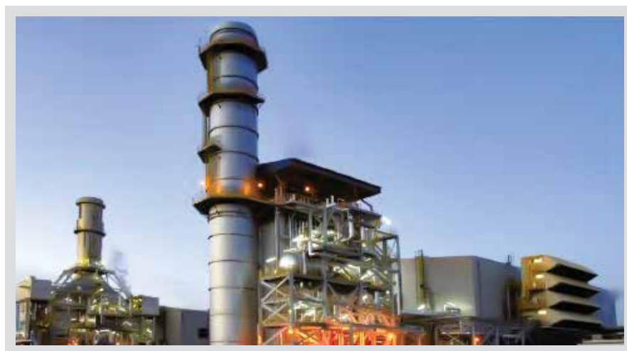
Gas Based Power Plant at Dahej SEZ, Bharuch, Gujarat.
