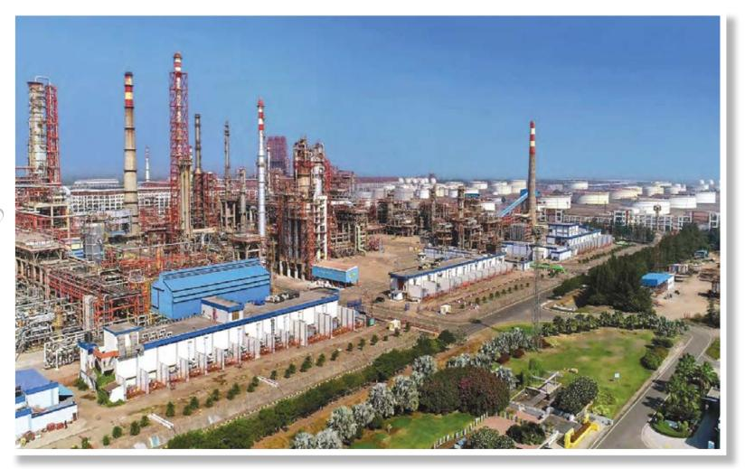
The 4,50,000 tonnes per annum polypropylene plant, a propylene recovery unit, revamp of existing FCC unit, LPG treatment unit and related offsites and utilities at the Vadinar refinery in Gujarat financed by SBI.
