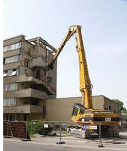
Fig 5. High reach excavator
